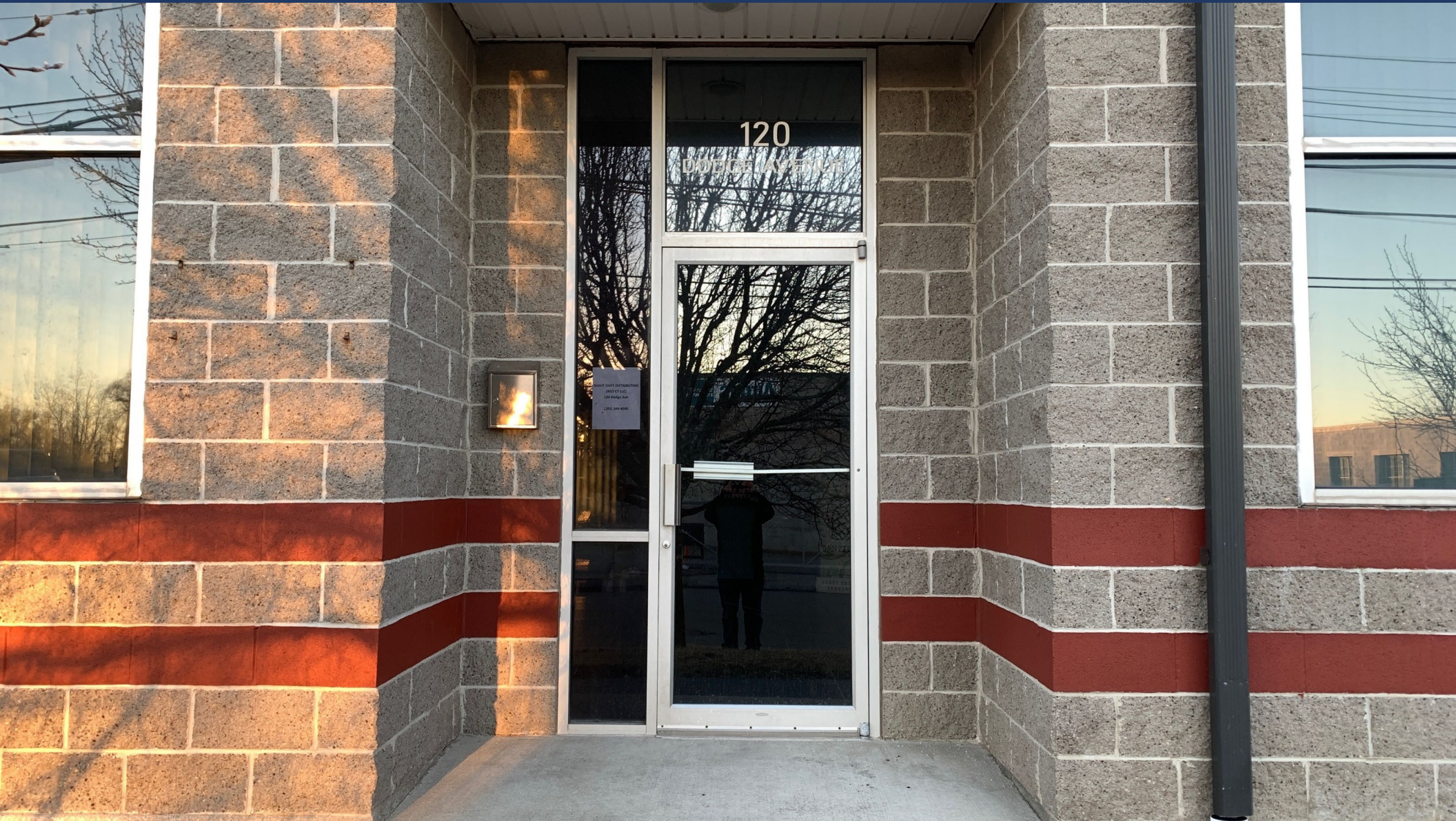
Front Entrance @ 120 Dodge Avenue
