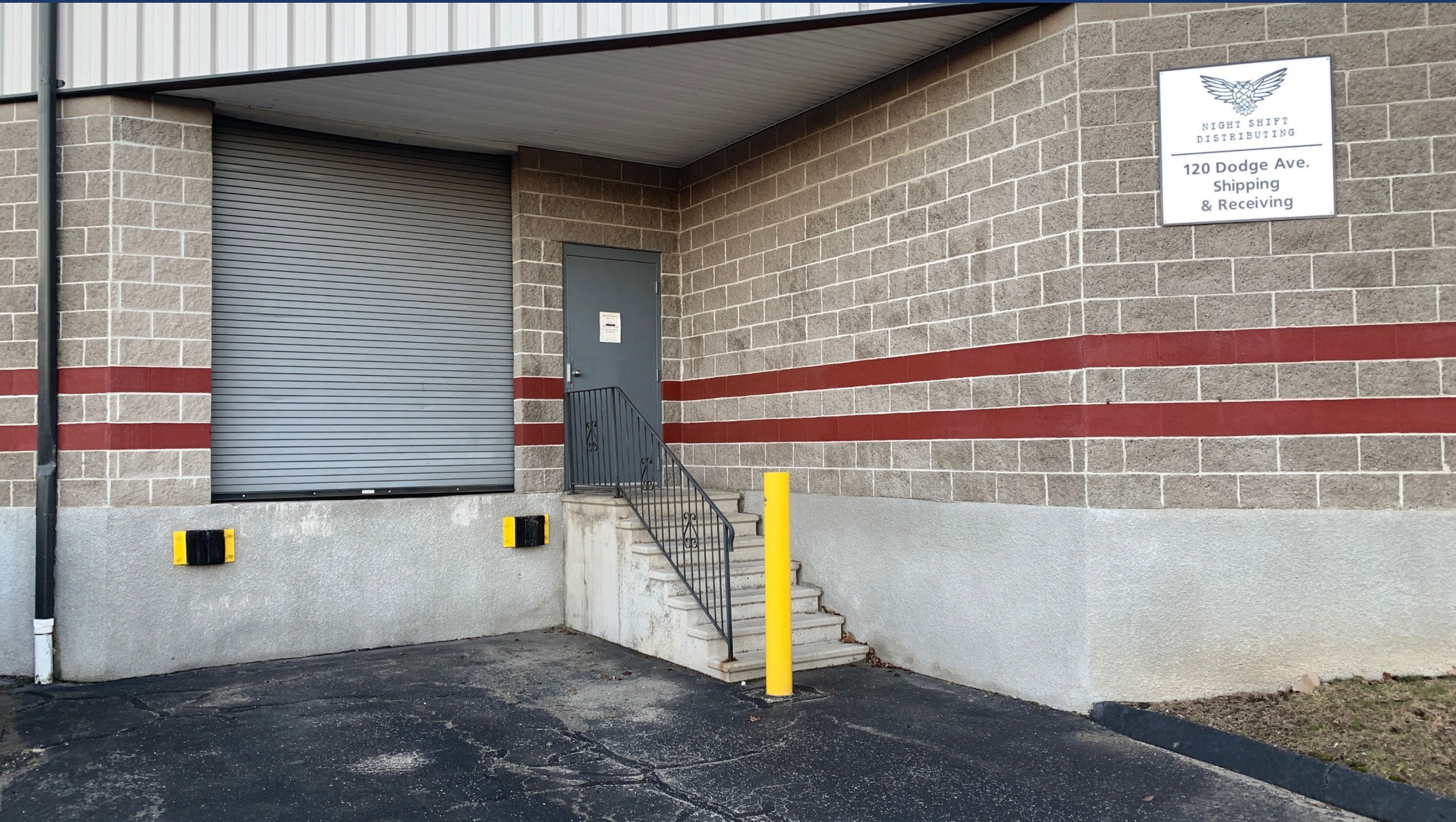
Loading Dock with Exit Door
